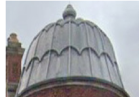
Lead roofing
