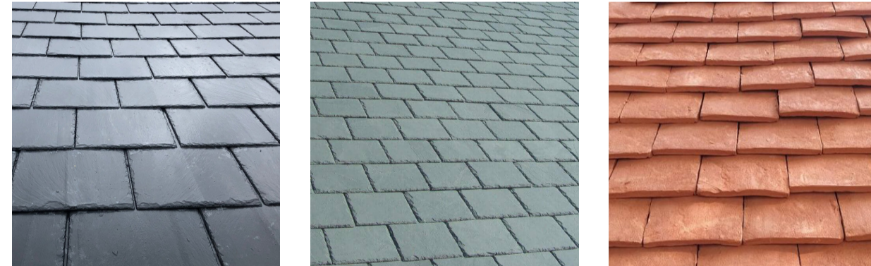
Tiled roofs in nearby context
